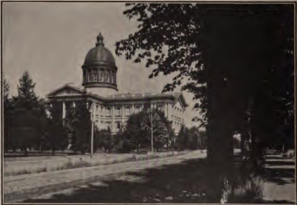
The capitol . . . is a stately and majestic building and the grounds about it are as beautiful as any in the United States
